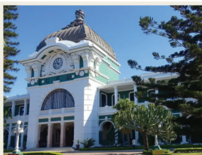
Maputo Railway Station
